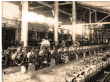
Inside of the Tobata Casting Factory
