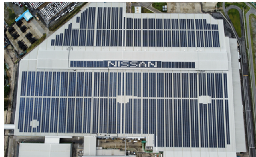
5.5 MW of solar power generation at the Thailand Plant
