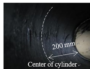
(c) Tank No.2 (Hoop layer from inner side).
