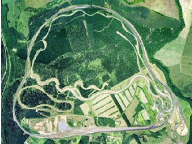
Fig. 2 PG of Nissan's Rikubetsu Proving Ground (Hokkaido)
