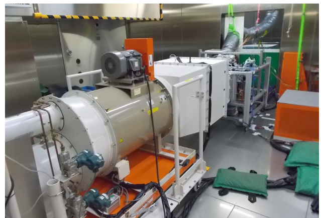
Fig. 5 Air-conditioner cycle bench test equipment
