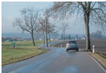
図-3 欧州の道幅が狭い郊外路 Fig. 3 Narrow country road in Europe
